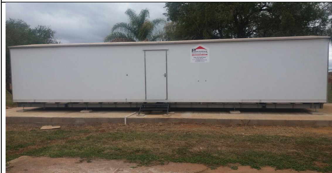
Image 1: Disaster Management Building
